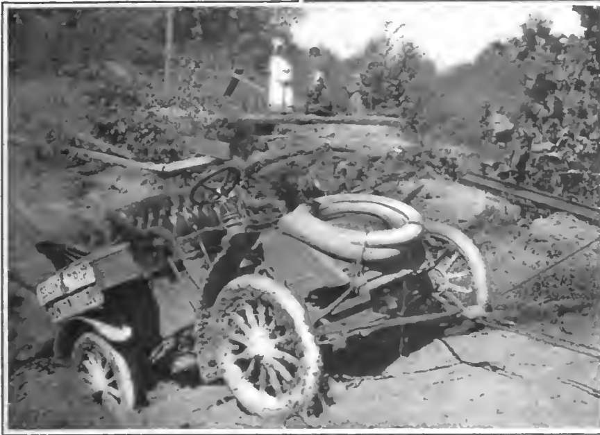
GETTING AROUND A WASHED OUT BRIDGE IN ILLINOIS WITH BLOCK AND TACKLE.
